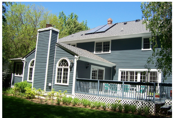
Solar hot water heating
