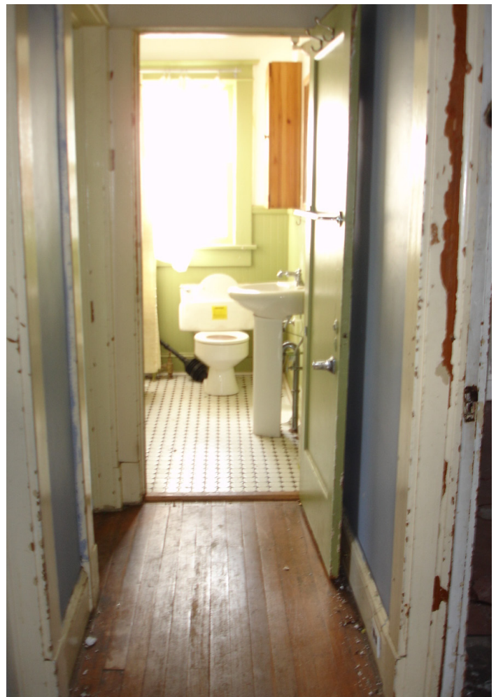
Upstairs bathroom before
