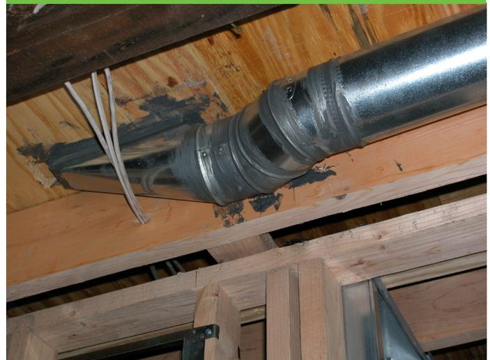
Ducts sealed with mastic
