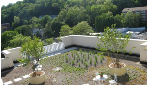
Figure 2 - The Geraldine R. Dodge Foundation headquarters green roof in Morristown, NJ (Source: Wild New Jersey )
