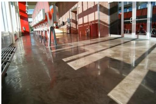
Figure 3 – Stained concrete floor (source: Rutgers Center for Green Building)
